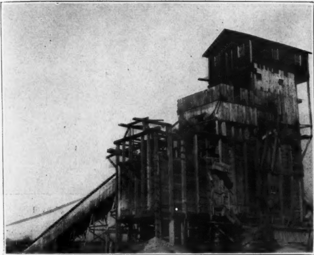
View of Screening Plant Showing Conveyor from Grizzlies and Crusher
